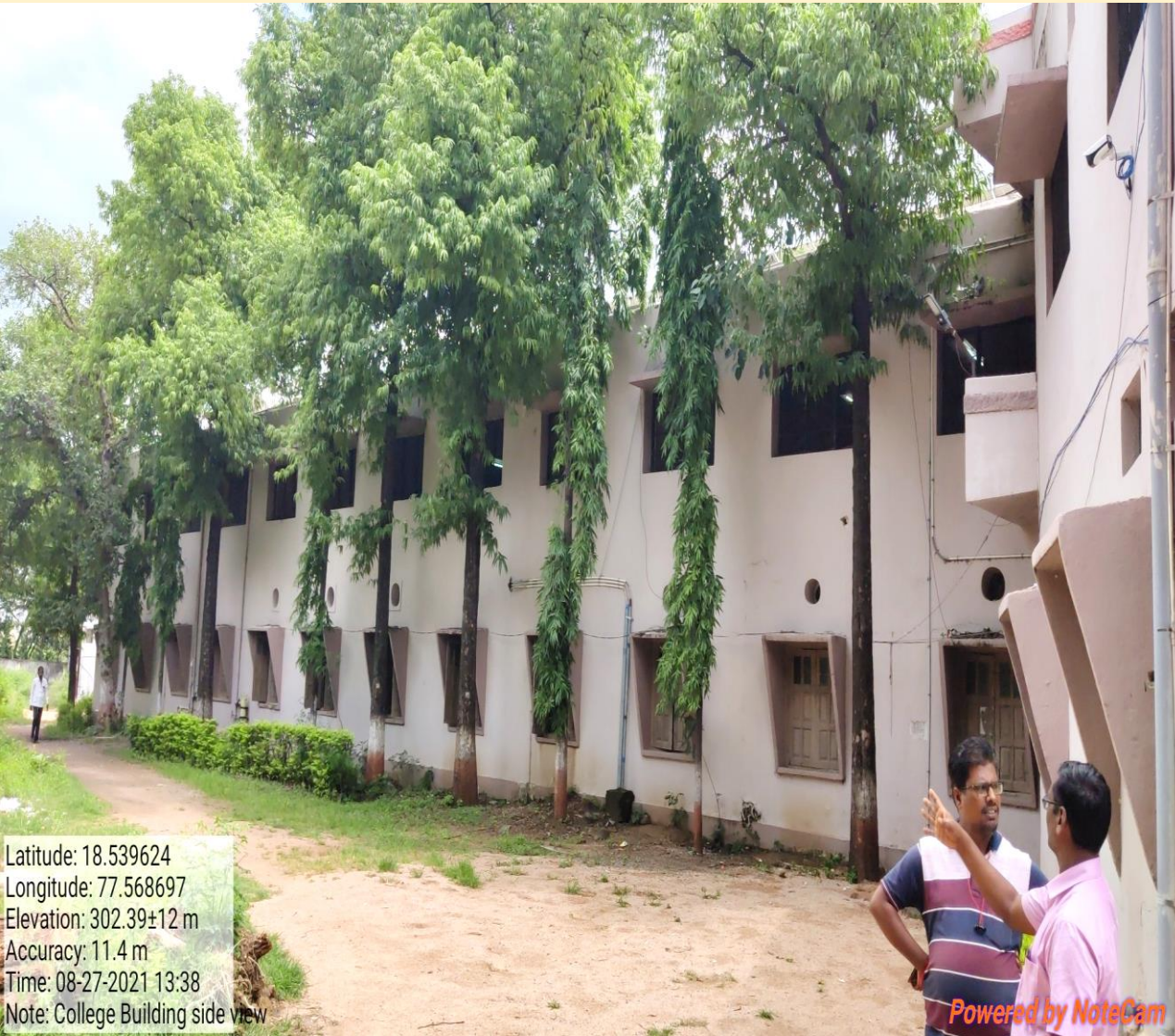
Building Left Side View
